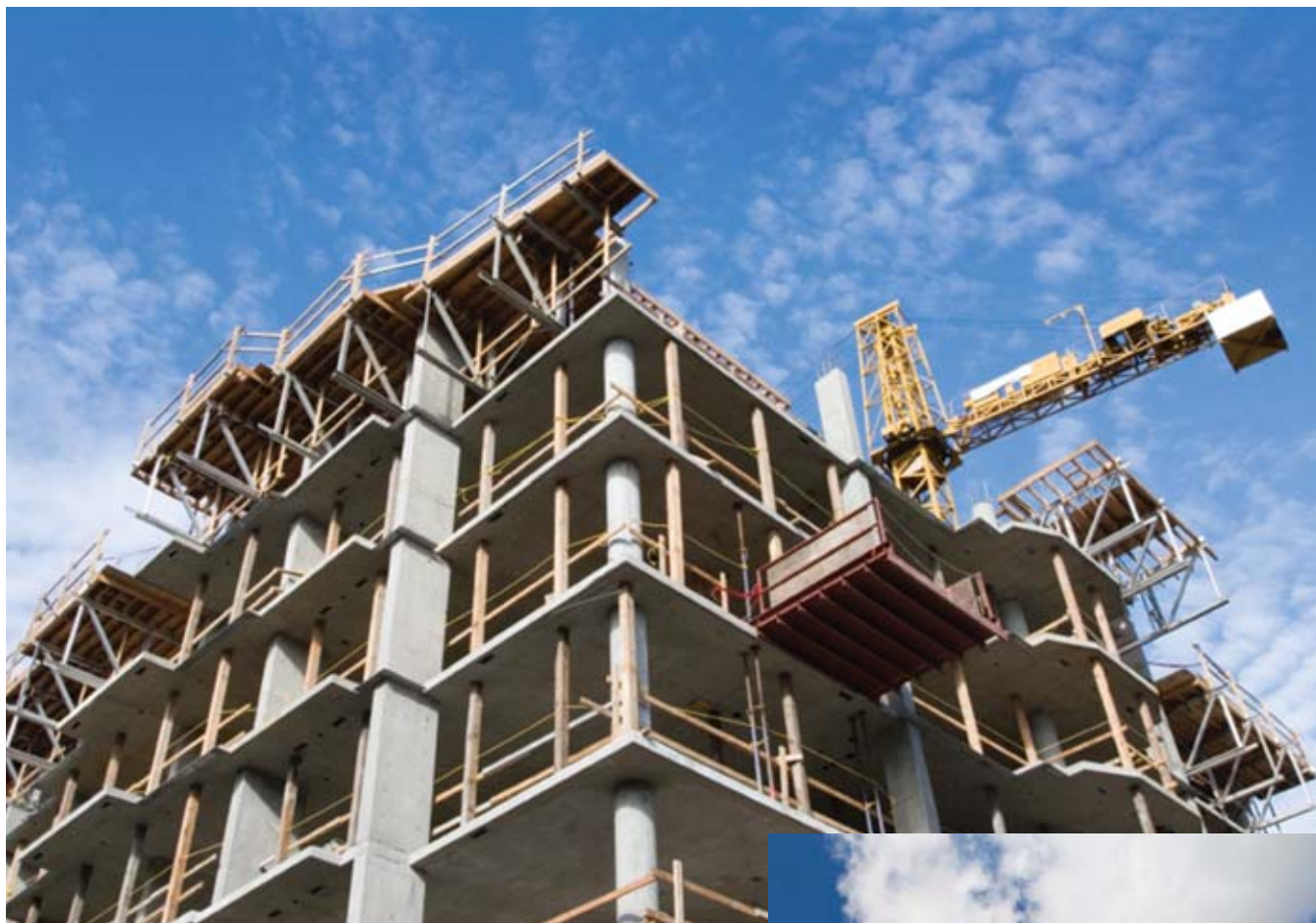
Construction Elevator Emergency Stops
